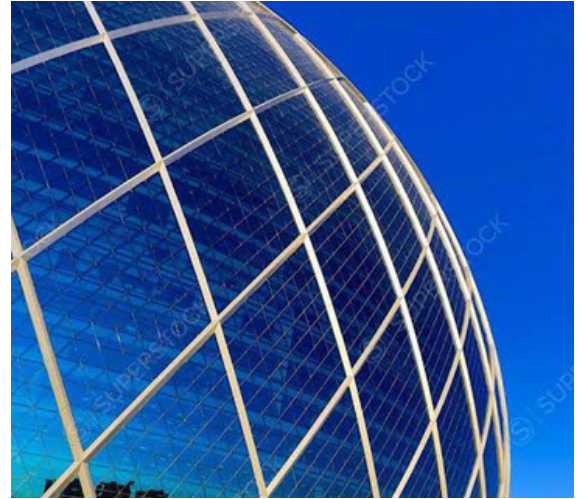
Al Raha Company Building
